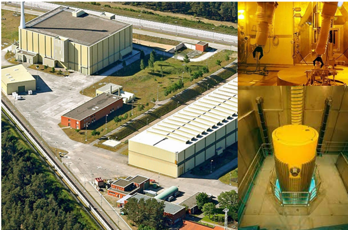
Figure 8-2: German pilot post-conditioning plant at the Gorleben site (left), view into the fuel handling cell (right above) and buffer storage POLLUX® cask (right below), based on (BGZ, 2021)
